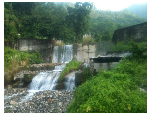
Figures: Different mitigating structures for debris flow across N-M Highway(Picture Taken 27 th September, 2014)
